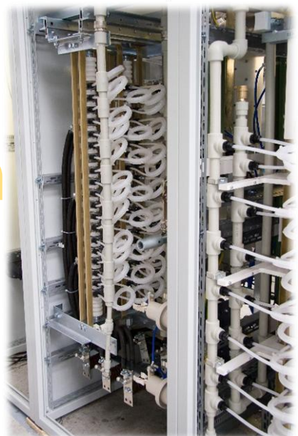
Image courtesy of CKD Elektrotechnika
